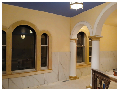
Chapel under construction
