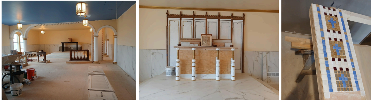
Chapel construction under way!
